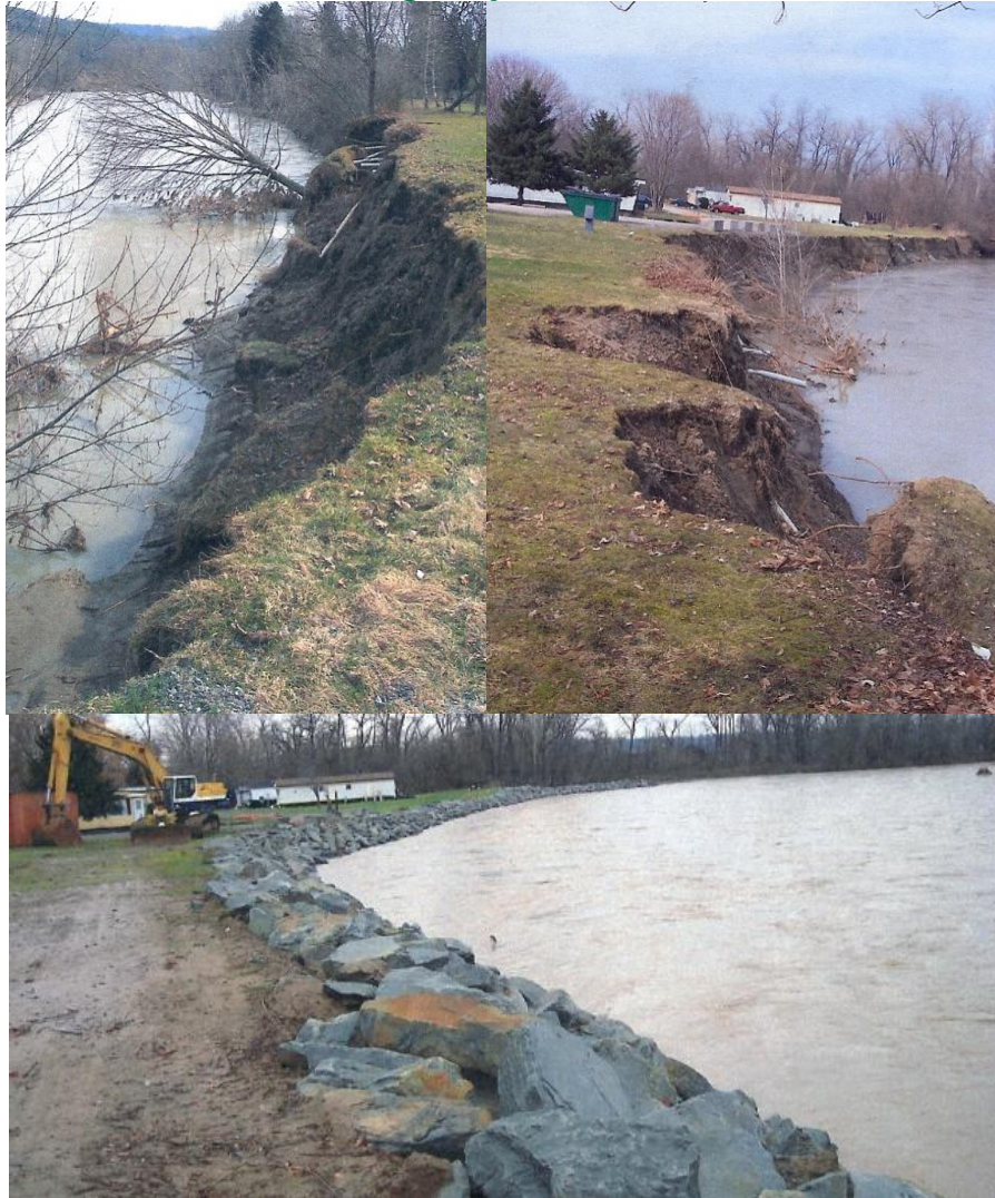
Before (top two photos) and After (at high water)(bottom photo): Photographs courtesy of Keith Folts
